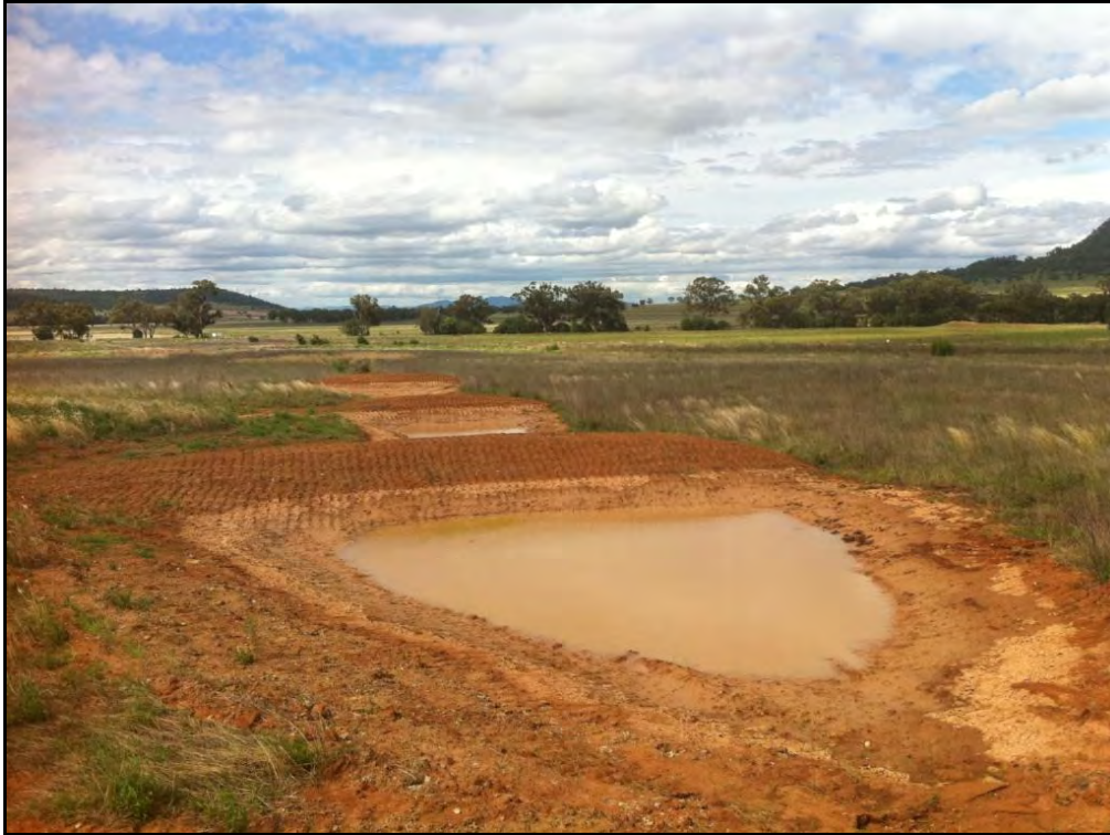
Plate 1 – Newly constructed sediment traps 30/11/2011
