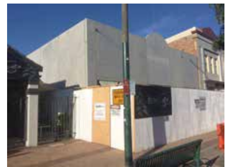
View from the outside
