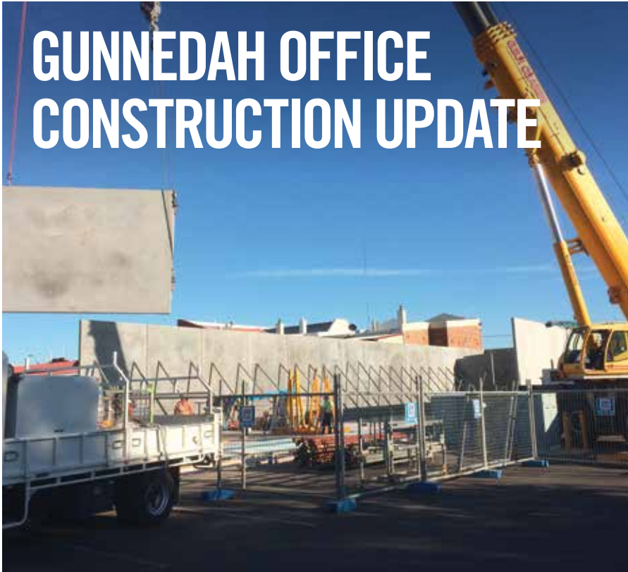
Walls going up
