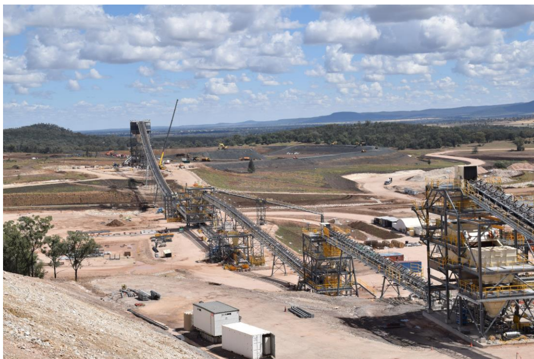
By-pass line from the ROM stockpile to the train loadout bin
