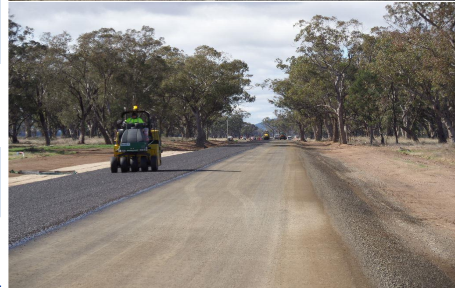
Road improvement under VPA with the local council
